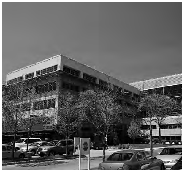
The fifth floor addition at Glenbrook Hospital is scheduled to open before the end of the year.
